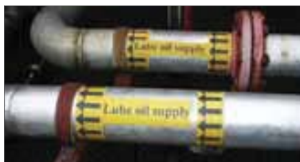
Pipe markers help describe pipe contents and direction-of-flow.
